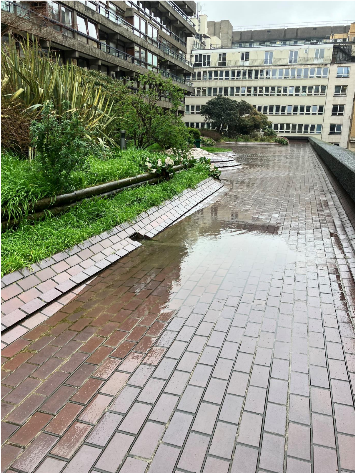
Image 3: The northern side of the Podium, showing pooling in rainfall events.
